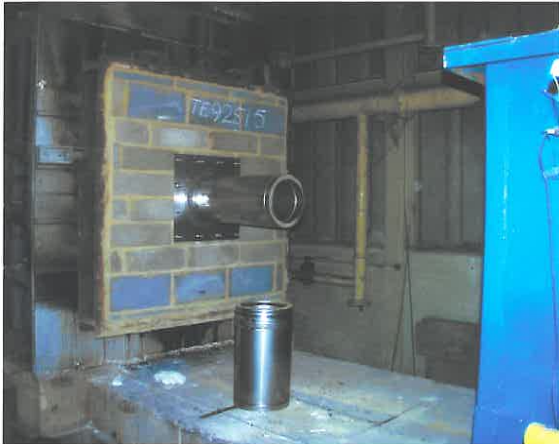
Plate 2 Detail of unexposed face of seal and chimney sections – MF100 (in place) and MF50 (free standing)
