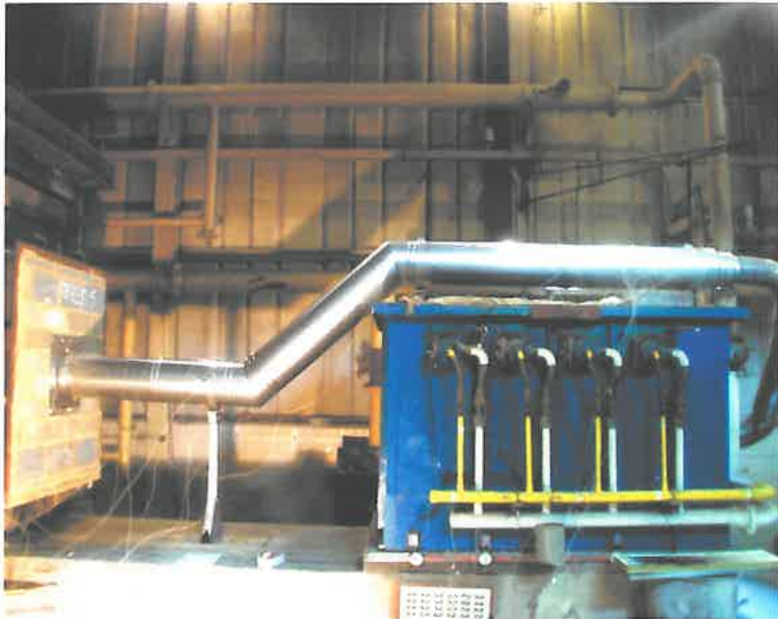
Plate 3 Chimney and penetration seal outside furnace before test
